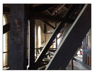
Its wooden frame could not be replicated today because there are no longer oaks tall enough. It's clad with a lead roof, and whenever it leaked more lead was added, until it became too heavy and had to be recovered
